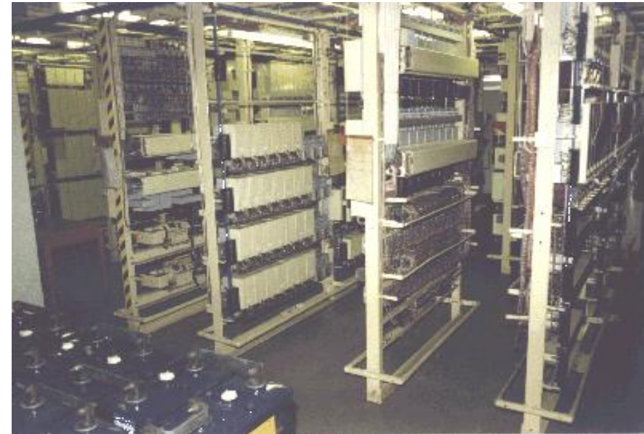
Automatic switching exchange
